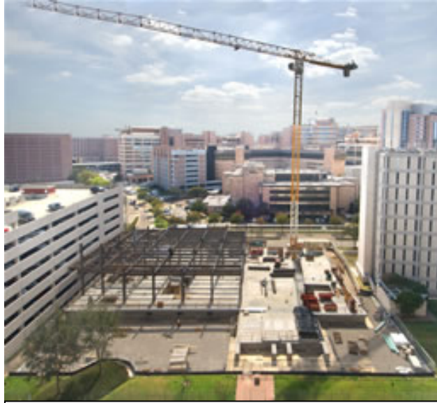
Figure 1: Tower under construction (3-1-06)
